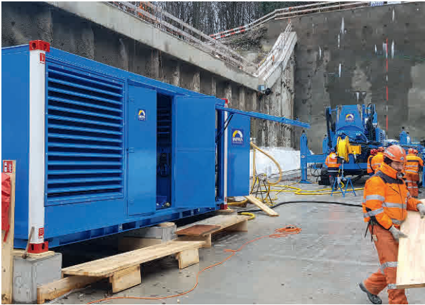
12 Pompe haute pression – 500 kW High-pressure pump – 500 kW
