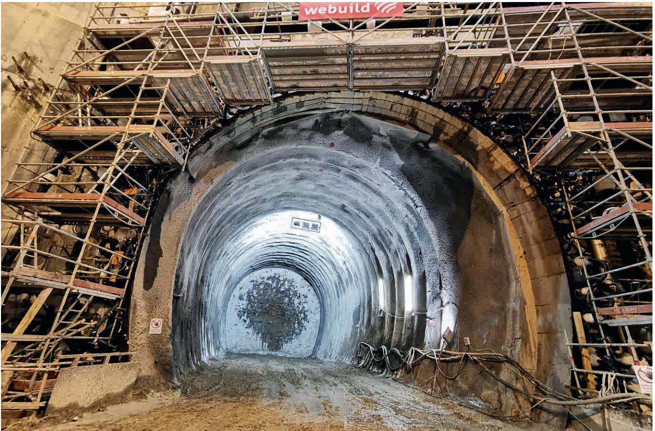
12 Scavo del terreno congelato Excavation of the frozen ground
