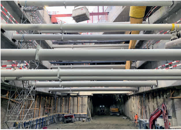
3 Aushubetappe 6, Deckelbau Eilgut Excavation stage 6, Eilgut cut-and-cover construction
