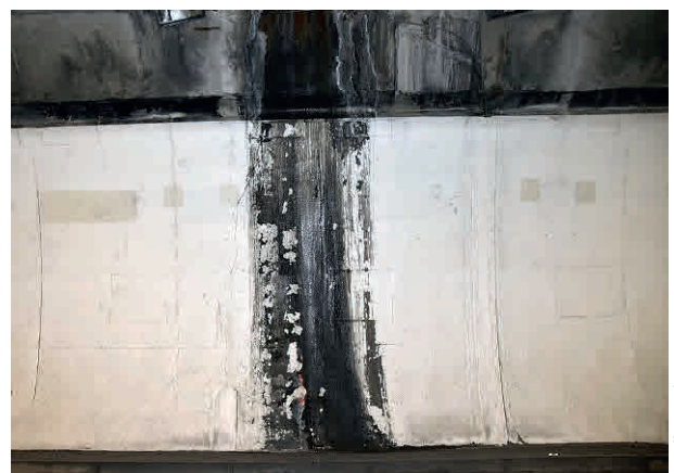
5 Wasserführende Risse, Strassentunnel Water-bearing cracks, road tunnel
