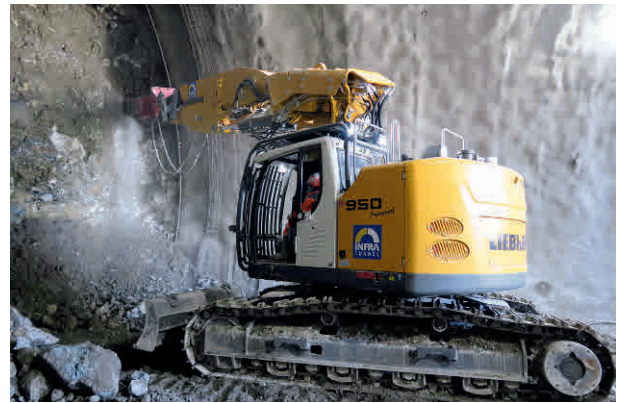
16 Excavation à la pelle hydraulique tunnel et brise-roche 3 500 kg. Excavation via hydraulic tunnel excavator and 3,500 kg rock breaker
