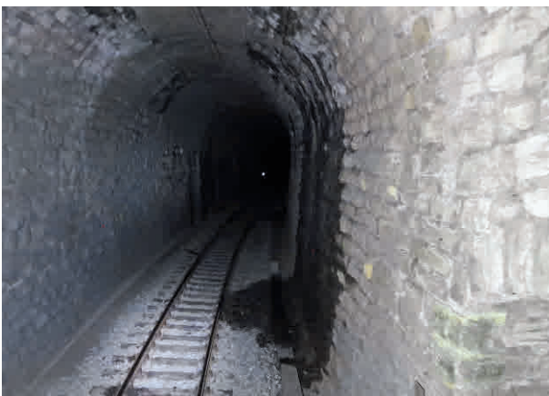
1 Feucht- und Tropfstellen, Bahntunnel Damp patches and dripping points, railway tunnel
