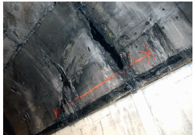
4 Wasserführende Risse, Strassentunnel Water-bearing cracks, road tunnel
