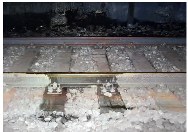
2 Tropfstelle, Bahntunnel Dripping point, railway tunnel
