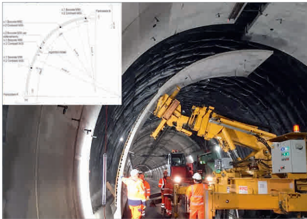
9 Montage der Predalles-Elemente Installation of the predalles elements
