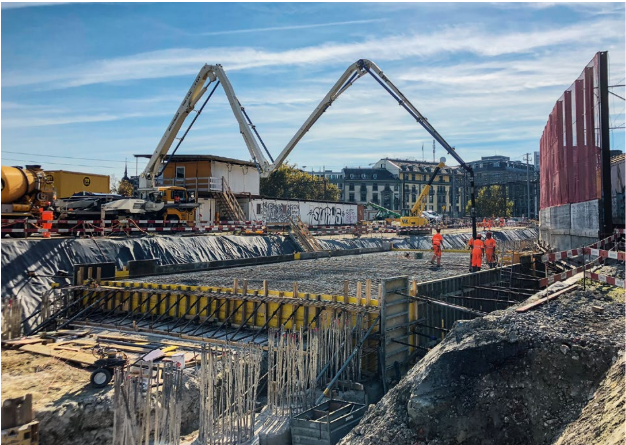
19 Eilgutareal – Betonierarbeiten Deckel (Blickrichtung Hauptbahnhof Bern) Eilgutareal – concreting works for cover (looking towards Bern Central Station)
