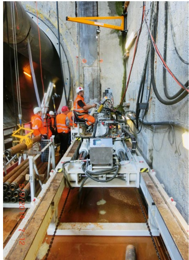
18 Probebohrungen in Berlin Test holes in Berlin
