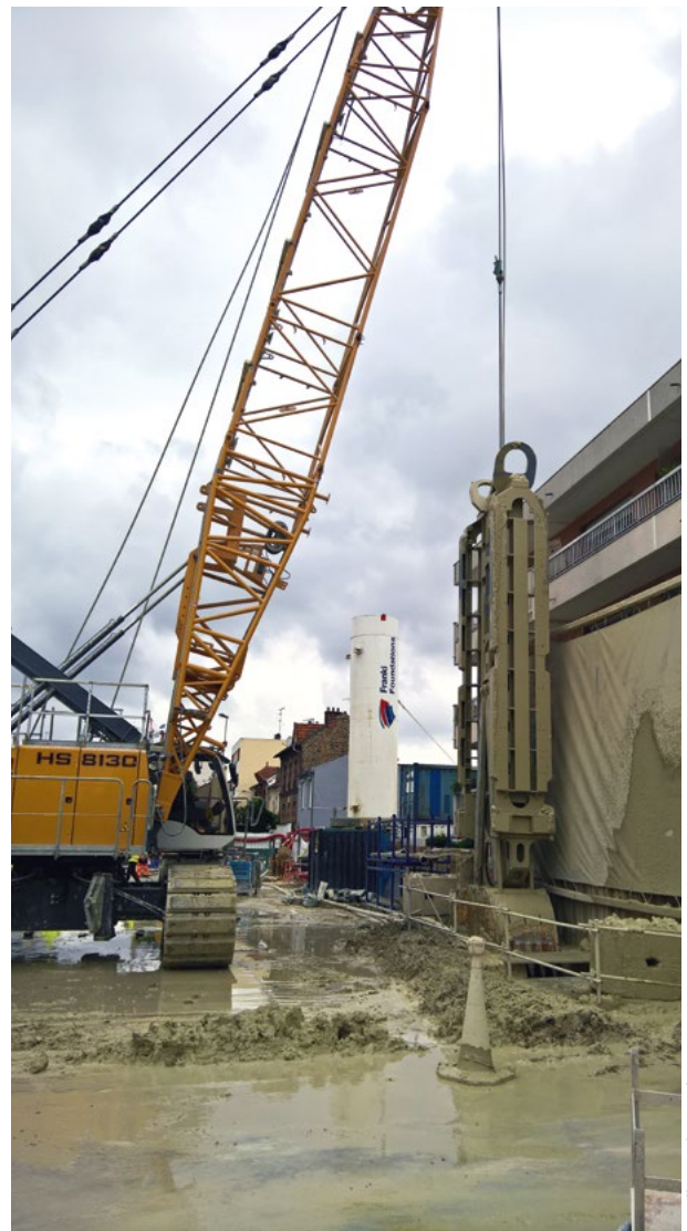
11 Station «Hôpital», Erstellung Schlitzwände “Hôpital” station, preparation of diaphragm walls
