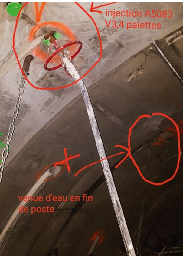
11 Premixed grout injection in zone A with worm pump and type of injection lance used
