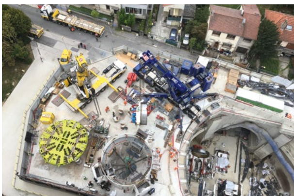
6 Startschacht/Montage TVM Starting shaft/assembly TVM
