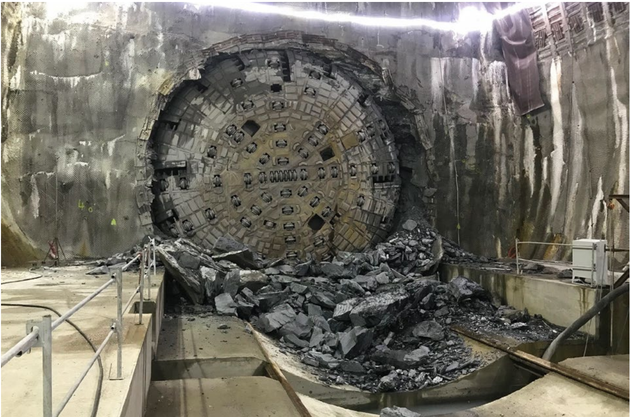
13 TBM breakthrough in La Praz
