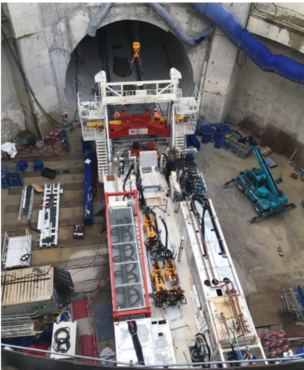
22 Montage TVM Startschacht TBM assembly access shaft
