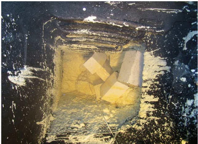
4 Additional coring with an external drill machine installed on CB and a cutterhead arm filled by expansive resin and polystyrene blocks
