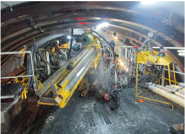
4 Additional coring with an external drill machine installed on CB and a cutterhead arm filled by expansive resin and polystyrene blocks
