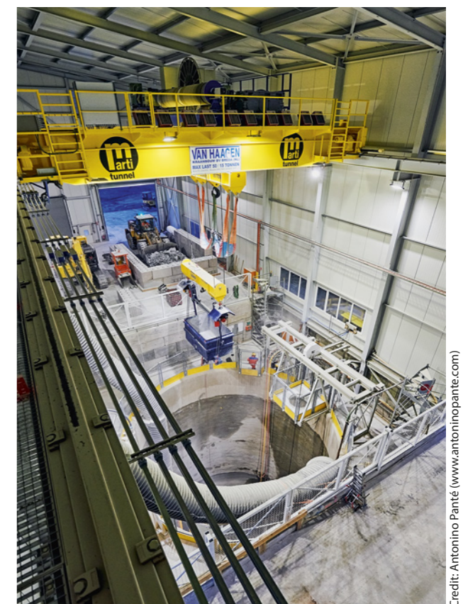
7 Shaft hall at Point 1
