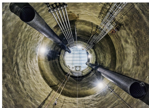
5 Rock support of Point 1 shaft
