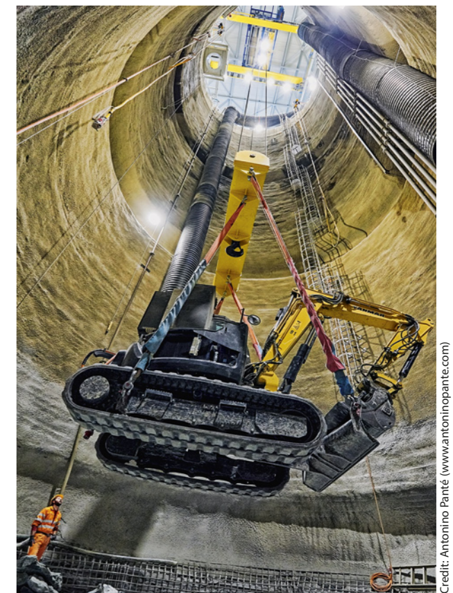
6 Shaft excavation at Point 1
