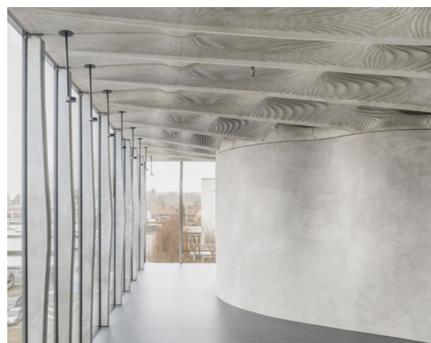
4 (left) The DFab House, a digitally planned house constructed using various digital fabrication techniques. (right) Concrete elements of the DFab House: right side, the Mesh Mould wall, made using the Mesh Mould process; top, the Smart Slab, made using 3D-printed formworks from the particle bed fusion process; left side, variable cross section facade mullions made using Smart Dynamic Casting.
