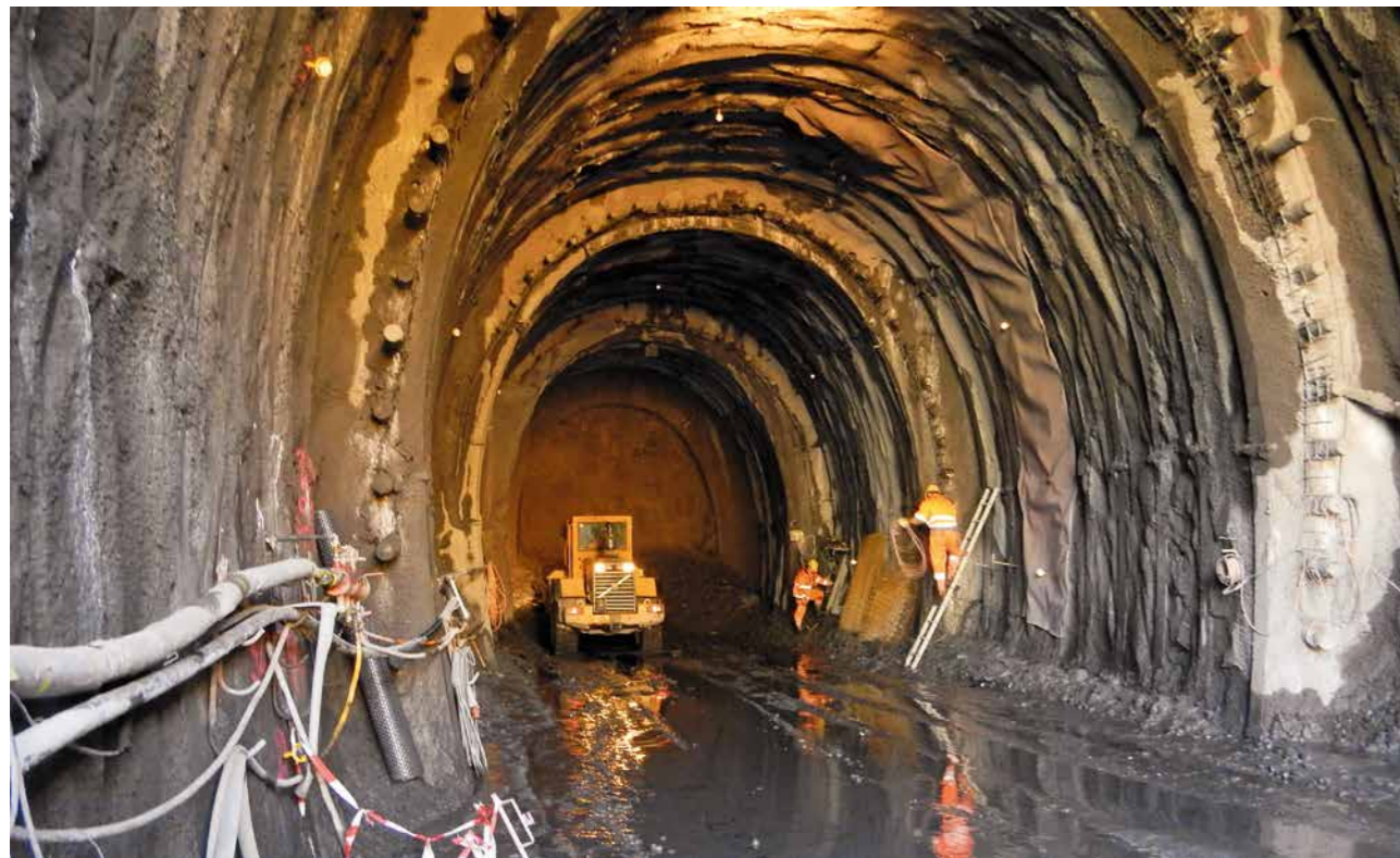
6 Rohrschirm Preda Preda pipe roof umbrella
