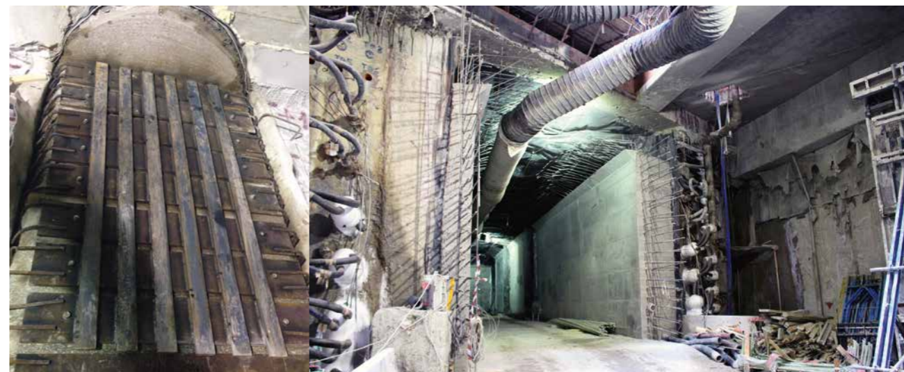
14 [a] The re-profiling foundation piles and [b] the permanent lining
