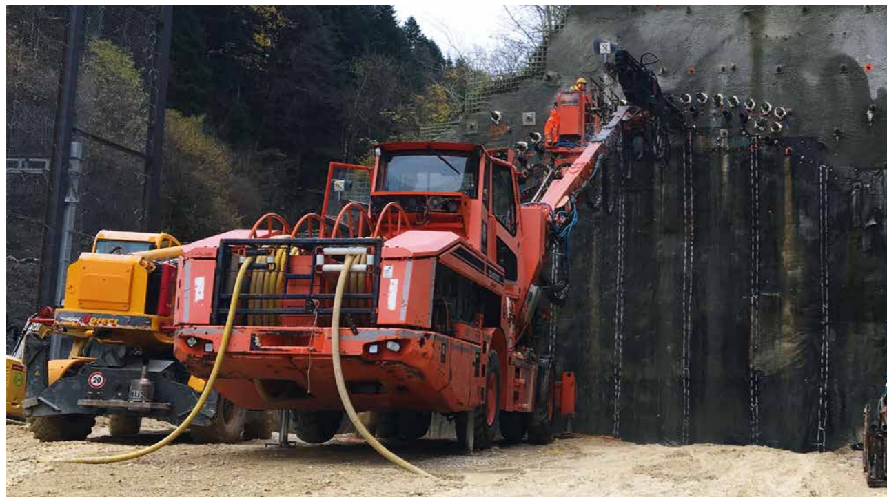
12 Bohren Dreifach-Rohrschirm Effingen Triple pipe umbrella drilling at Effingen
