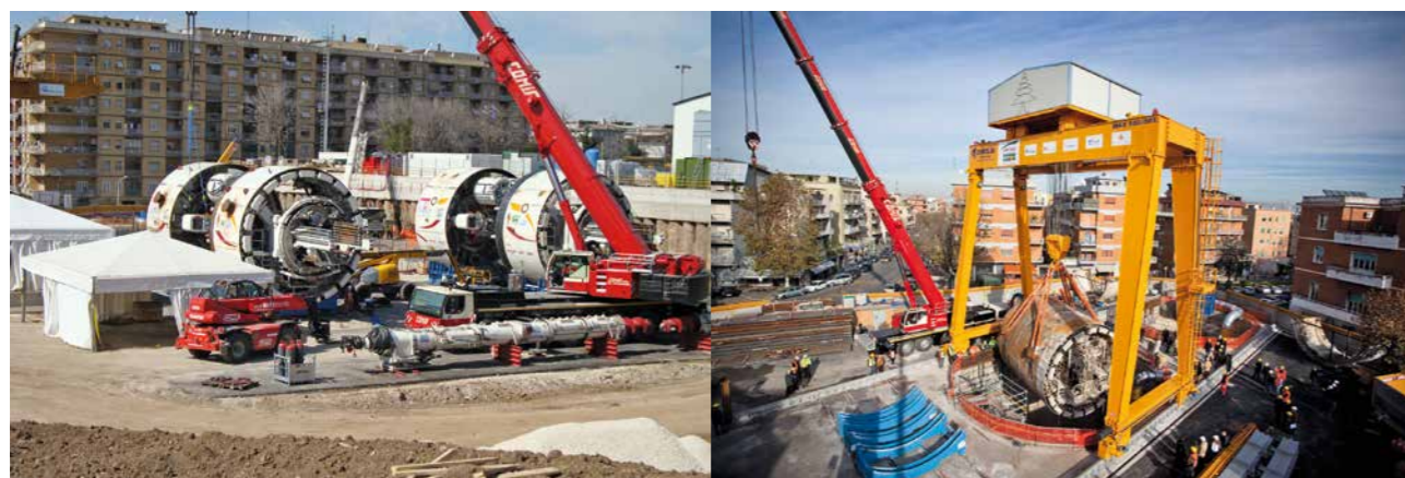
4 The two TBMs used for tunnel excavation and TBM handling
