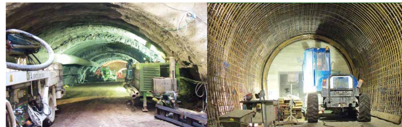
5 Tunnels excavated with the traditional open-face method
