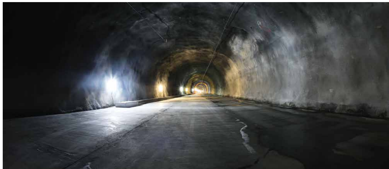
2 Bestehende Spurwechselkaverne Mitholz Südwest im Rohbautunnel West Existing track change cavern at Mitholz south-west in the unfinished west tunnel
