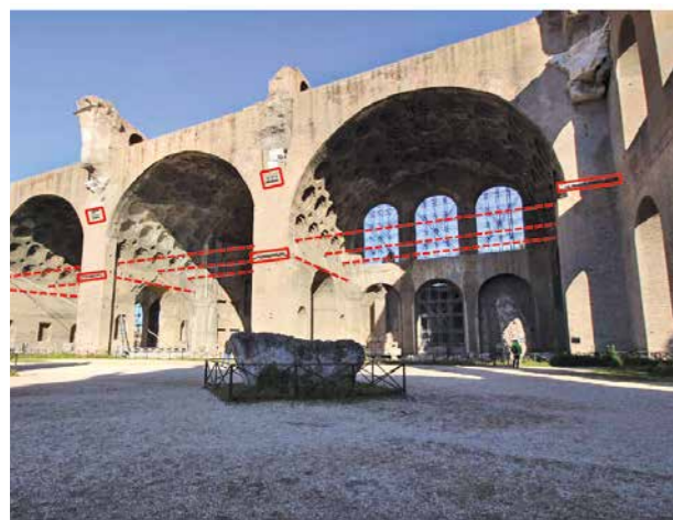
21 An internal view with the permanent structural reinforcements highlighted in red
