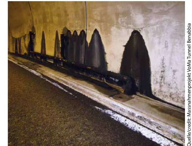
19 Wasserinfiltrationen, Tunnel Benabbia [14] Water infiltration, Benabbia Tunnel [14]
