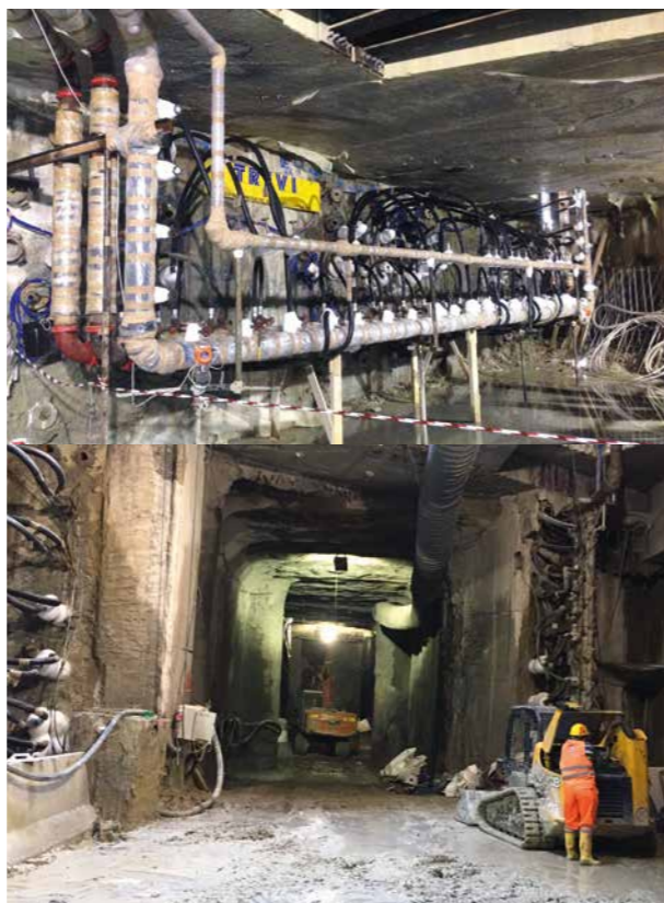
13 [a] Freezing pipes and [b] tunnel excavation
