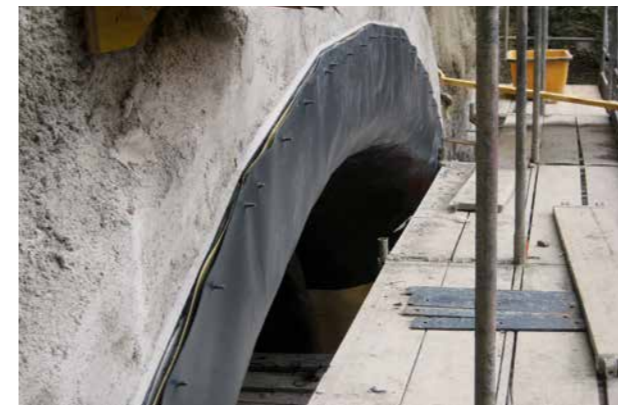
9 Abdichtungsübergang Tunnel-Tagbau (Portalwand) Sealing transition from tunnel to surface construction (portal wall)
