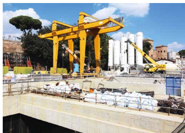
22 View of the shaft 3.3 worksite
