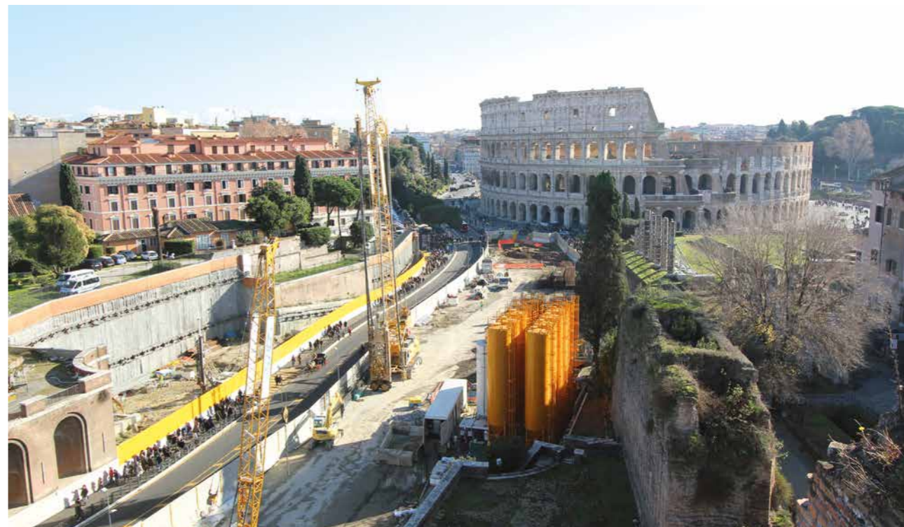
15 A view of the Fori Imperiali station construction site
