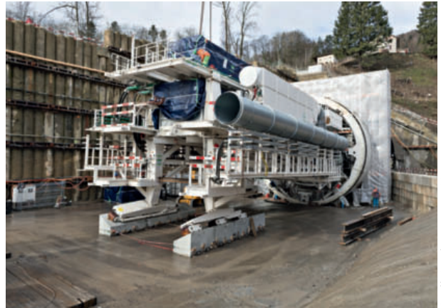
14 Montage TBM TBM assembly
