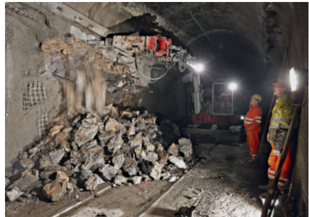
8 Charnadüratunnel, Gewölbeabbruch Charnadüra Tunnel, vault demolition
