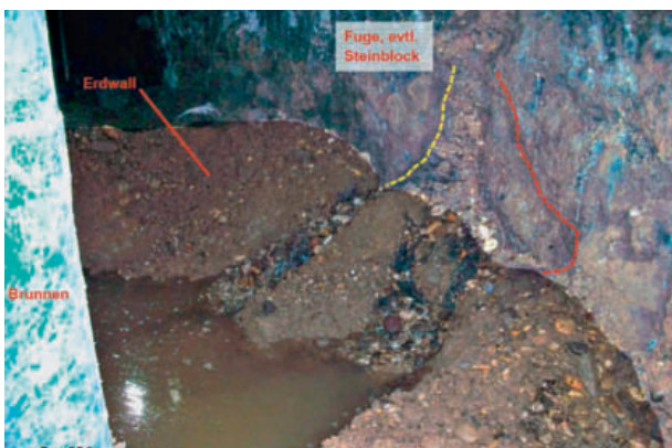
12 Wasserzutritte vor Fuge 10/11 am Unglückstag Ingress of water upstream of joint 10/11 on the day of the accident
