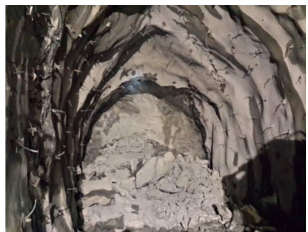
12 Rockburst event in the headrace tunnel
