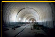
CEVA, Tunnel de Pinchat (GE)
