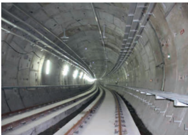
3 View of tunnel after works
