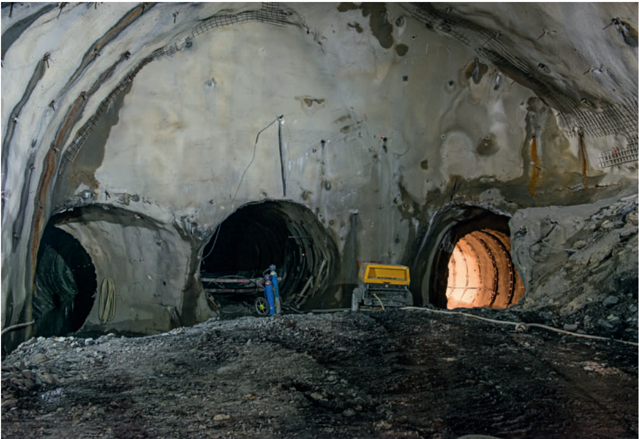
8 Widerlagerstollen links und rechts ab Tunnelmeter 1076,50 (Schutterstollen in der Mitte) Abutment tunnels to the left and right as from tm 1,076.50 (mucking tunnel at the centre)
