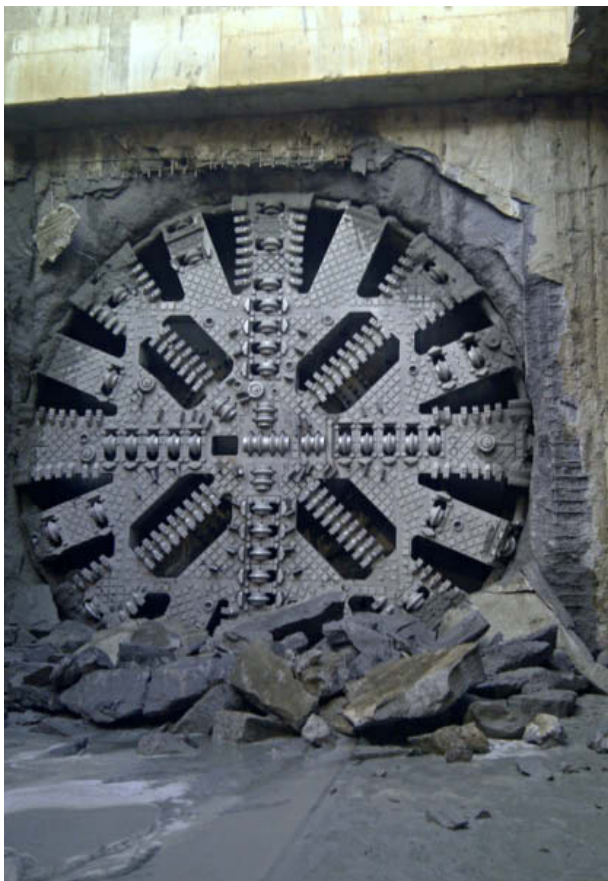
7 TBM breaking through into station
