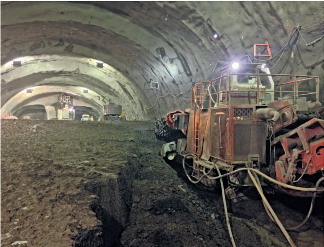
10 View of upper drifts at Lyon station
