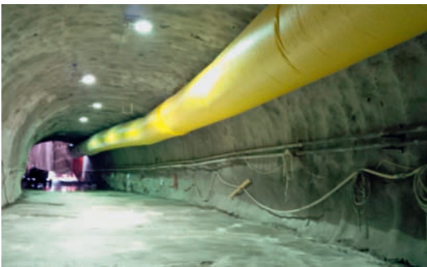
4 Running tunnel excavated with roadheader
