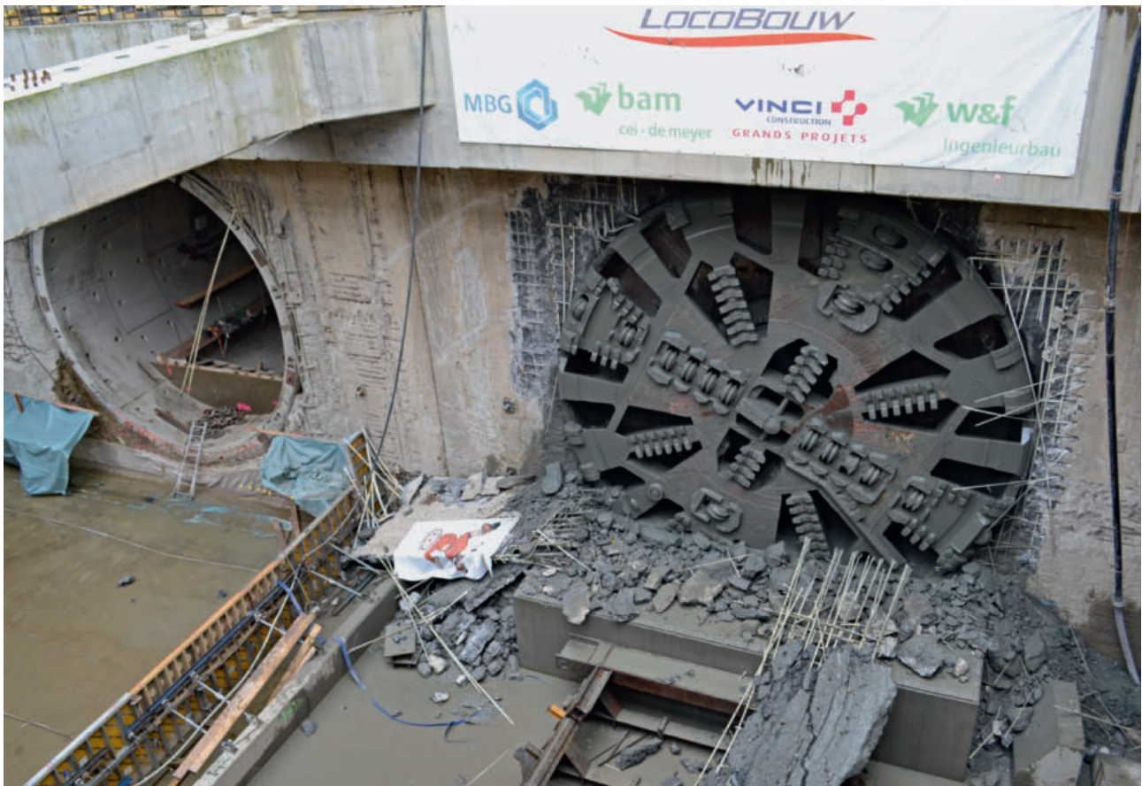
11 Ankunft TBM Nord (rechts) und Tunnel Süd (links) Arrival of north TBM (right) and the south tunnel (left)
