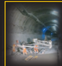
CEVA, Tunnel de Pinchat (GE)
