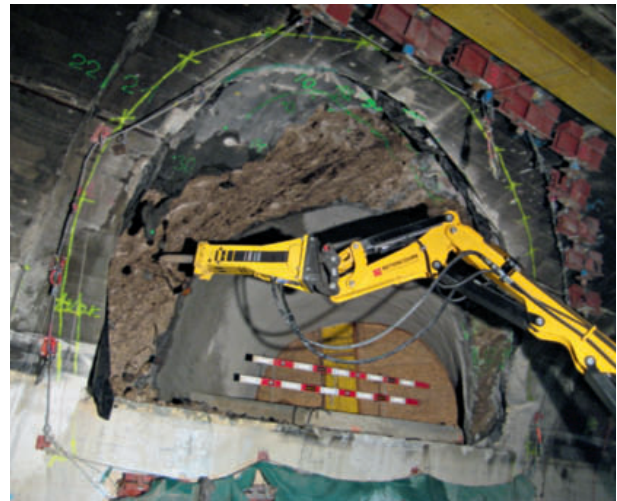
6 Abbau Querstollen A2-Tunnel Belchen Cross passage excavation A2 Belchen Tunnel
