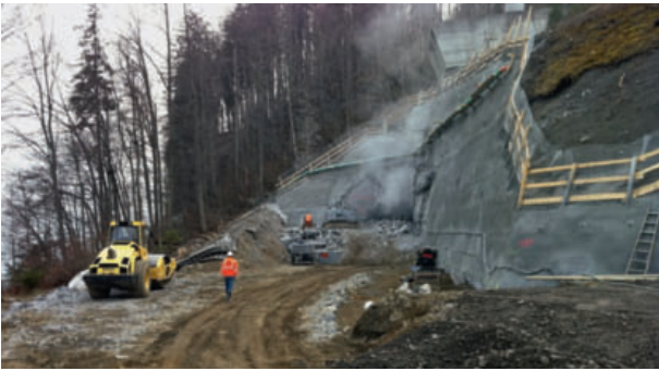
3 Voreinschnitt Giessbach West in Arbeit Giessbach West pre-cut under construction
