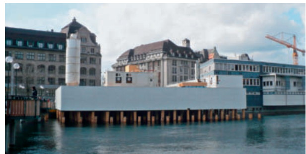
4 Installationsplattform Limmat Installation platform in the Limmat
