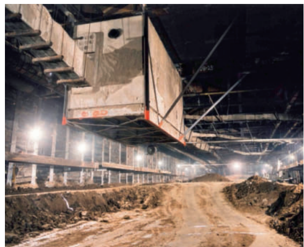
5 Utilities in operation under the slab
