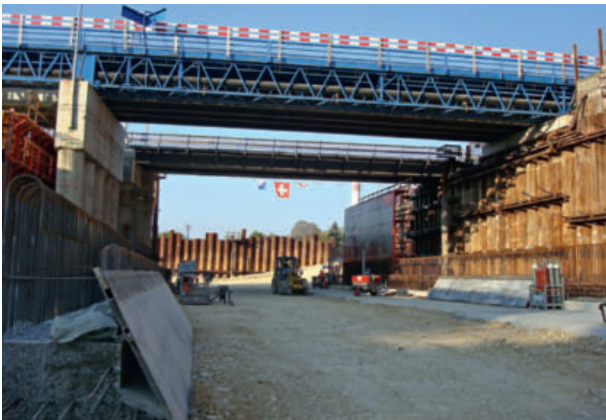
10 Bahnquerungen Ostast, Brüggmoos Railway crossings at the east branch, Brüggmoos
