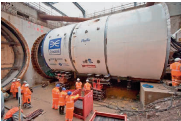
2 Royal Oak portal – main tunnel site
