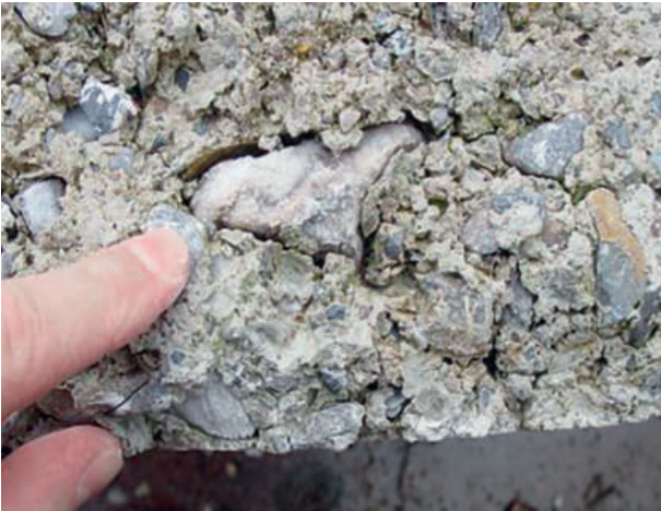
7 Risse in der Kontaktzone Gesteinskorn-Zementstein Cracking in the contact zone between aggregate particles and cement paste
