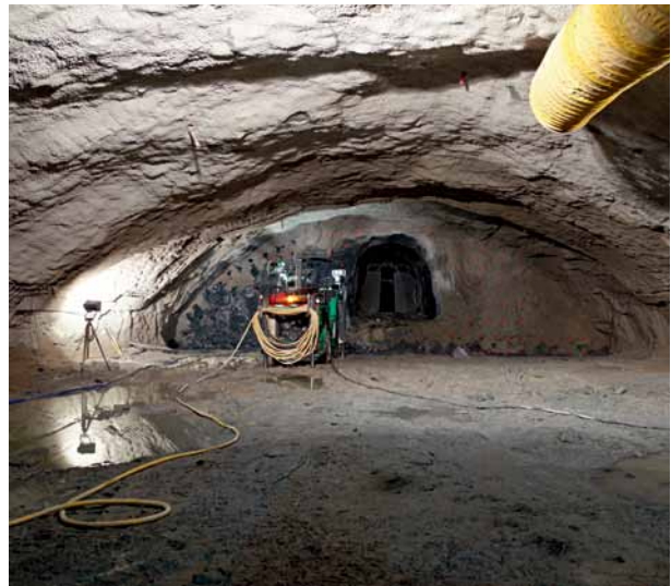
10 Caverne principale – Phase 1 des terrassements Main cavern – Phase 1 of the groundworks
