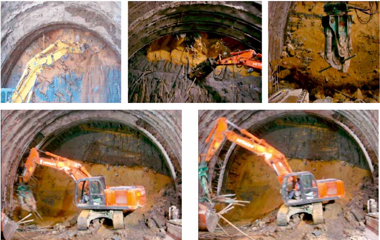
16 Excavation phase in Serra dell'Ospedale Tunnel
