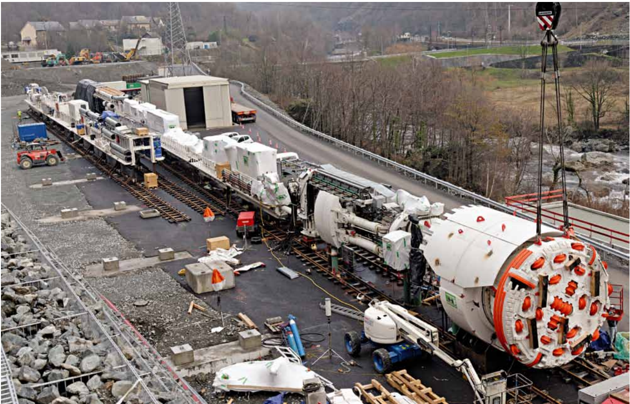
6 Montage sur plateforme du tunnelier aval: "Rosali" Mounting on the downstream tunnel boring machine platform: "Rosali"
