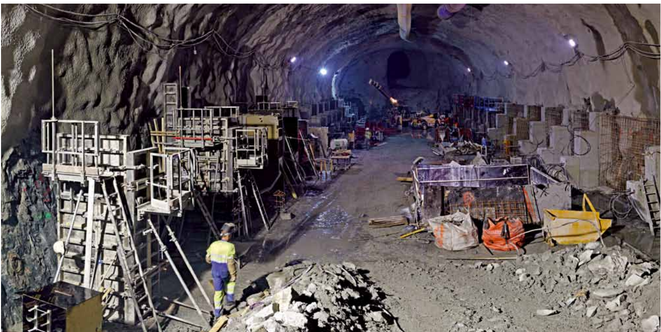
11 Caverne principale – Phase 2 des terrassements Main cavern – Phase 2 of the groundworks
