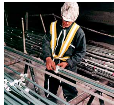
11 Example of the reinforcement element obtained with plate elements assembled around and injection pipe with "manchette". Shown on the right side is the assembly of the element directly on the job site
