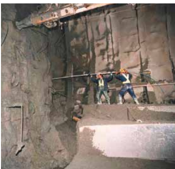
11 Example of the reinforcement element obtained with plate elements assembled around and injection pipe with "manchette". Shown on the right side is the assembly of the element directly on the job site
