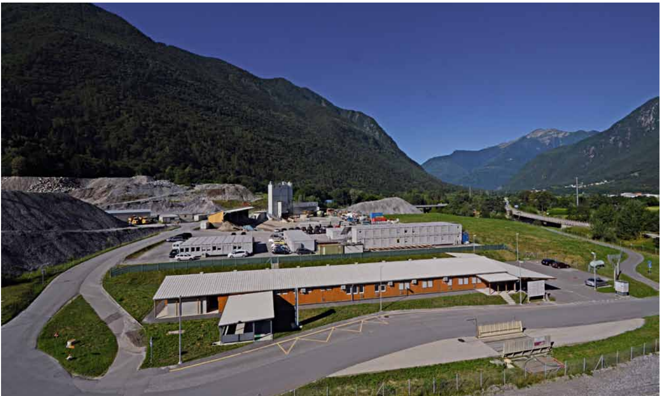
8 Baustelleninstallationen Construction site installations
