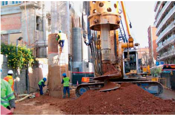
16 Pile excavation
