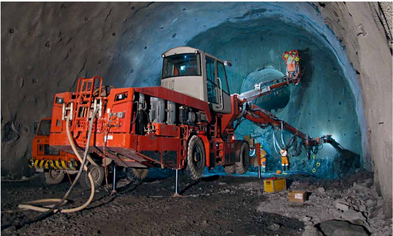
10 Blick in den Sprengvortrieb View of the drill & blast drive
