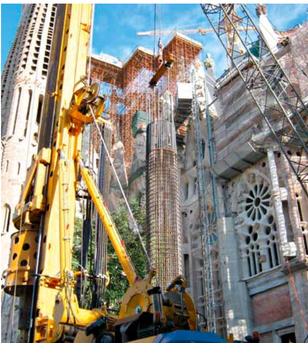
17 Pile wall construction
