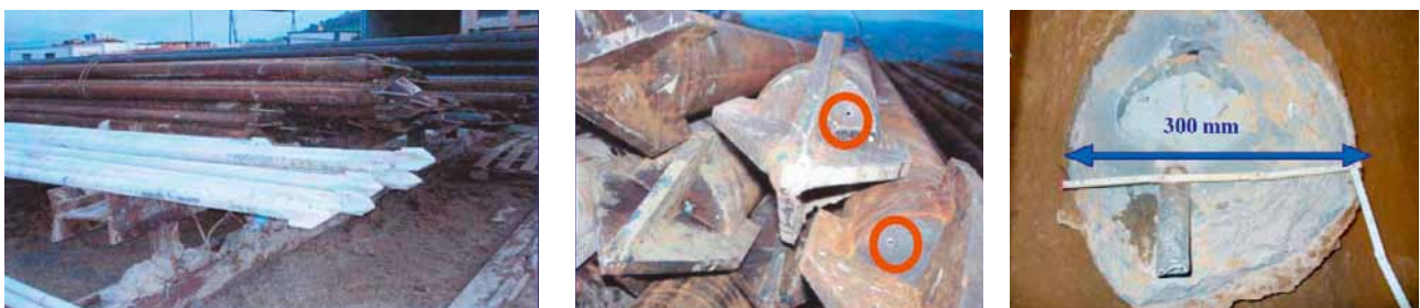
15 Detail of the steel pipe used in the Serra dell'Ospedale tunnel and view of the pipe after installation with the grout mix injection
