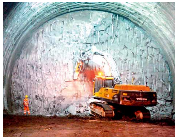
6 Tunnel face during excavation
