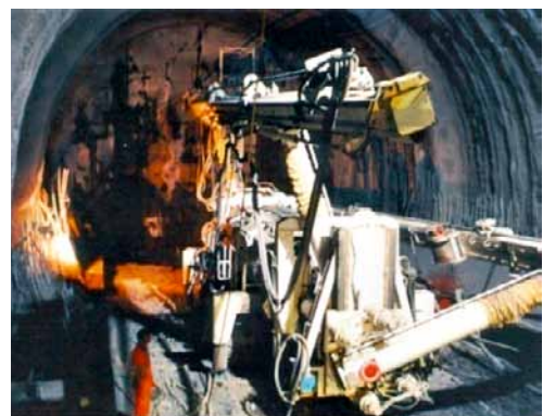
8 Example of a modern double boom machine (Trevi SM605 AV). Stroke: 24 m; radius of consolidation treatment at 0°: 3,600 to 6,600 mm; height from working level of slew ring rotation centres: 1,000 to 3,500 mm; max. distance from the tunnel face: 12 m; short boom to drill with inclinations: from 16° to 37°; max. power (2 separate motors): 349 kW (Source: TREVI)
