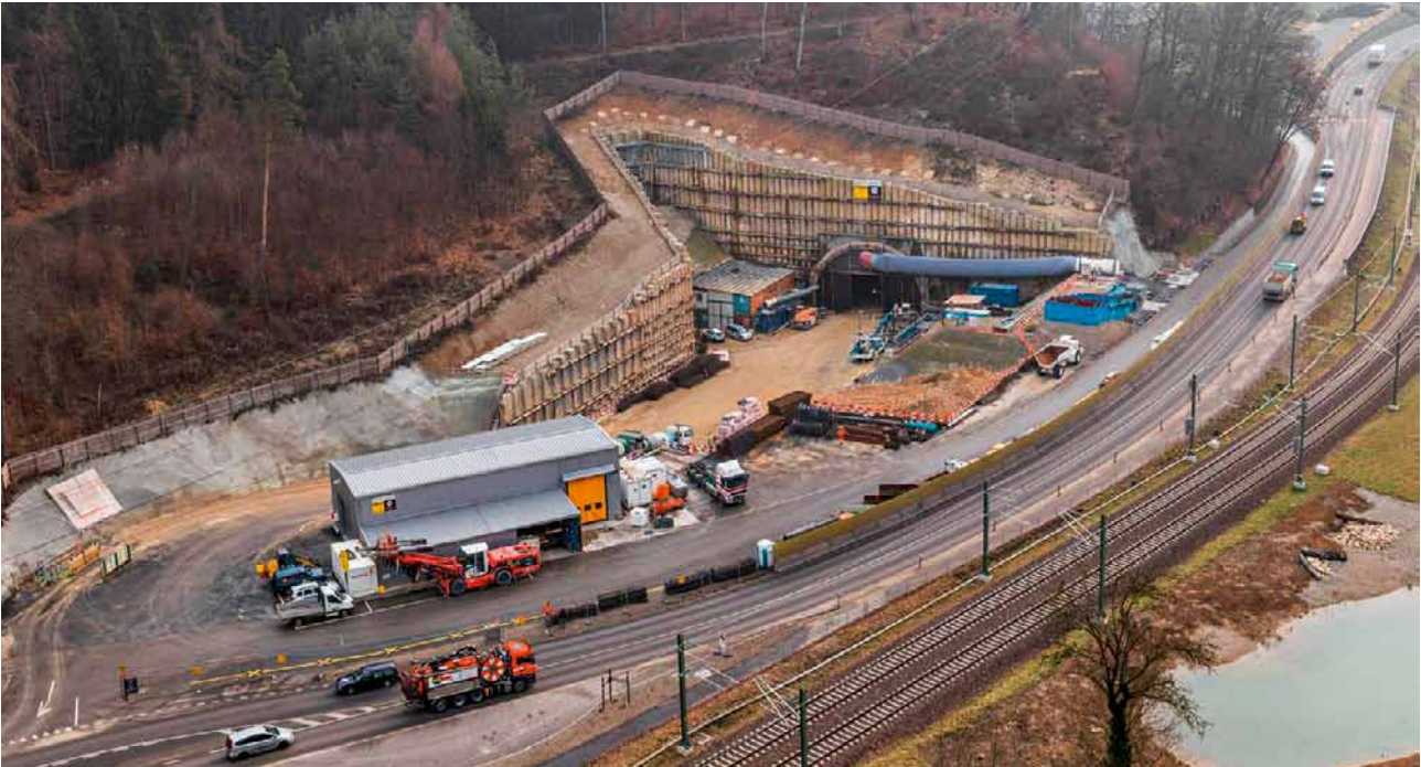
7 Installationsplatz Engi Engi installation yard
