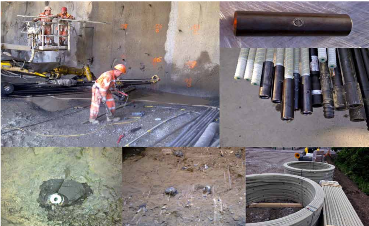
9 Boulon autoforeur GFK traditionnel Traditional self-drilling GFRP anchors
