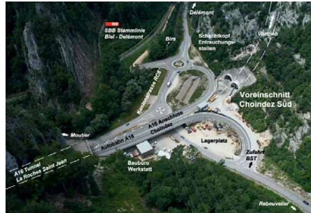
4 Situation am Portal Süd Situation at south portal
