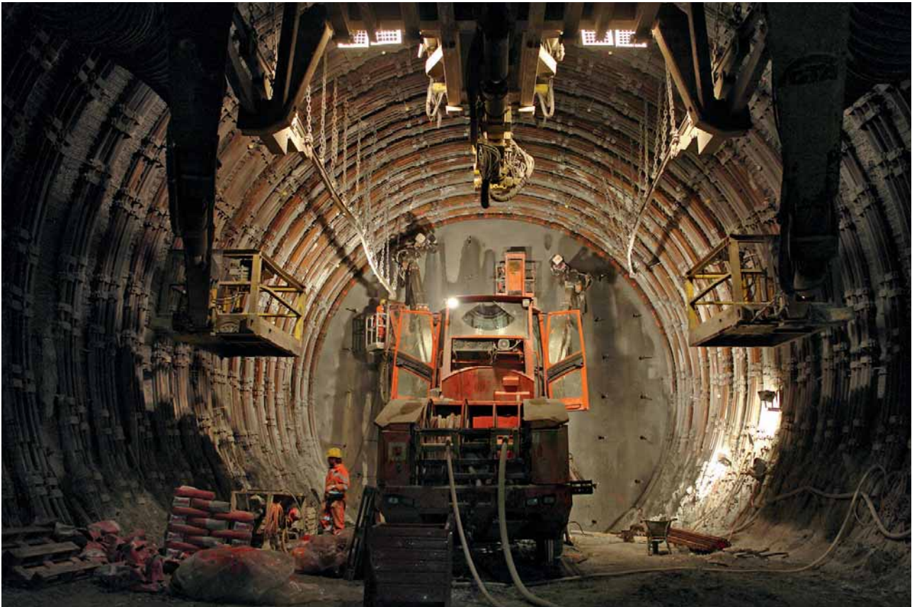
2 Sedrun – deformierbarer Stahleinbau TZM Nord Sedrun – TZM North deformable steel structure
