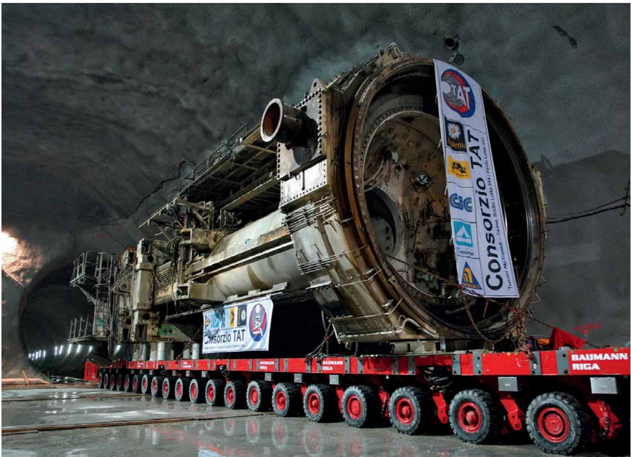
4 Faido – Zwischentransport TBM Faido – TBM interim transportation
