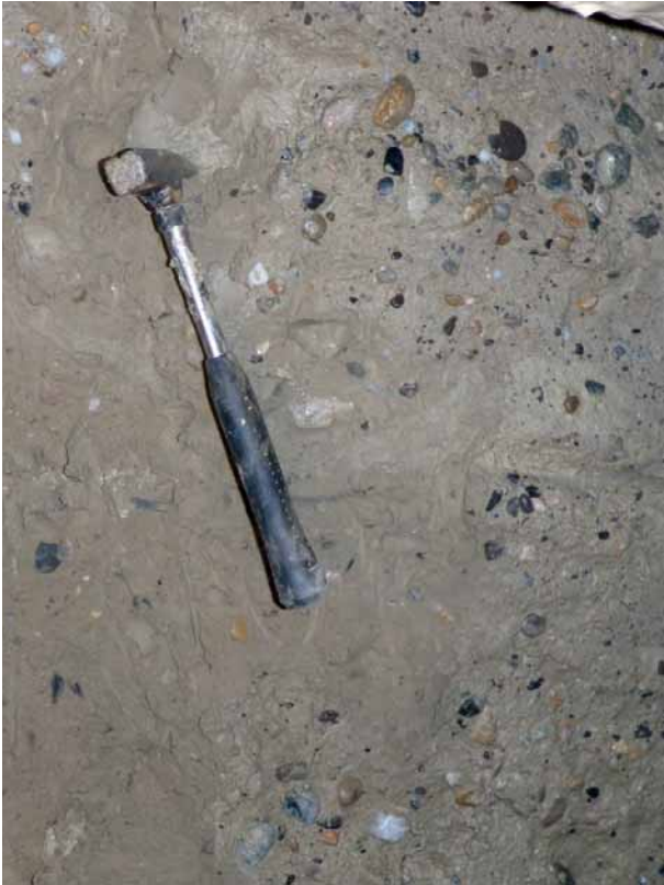
10 Filterkuchen an der Ortsbrust Filter cake at the face
