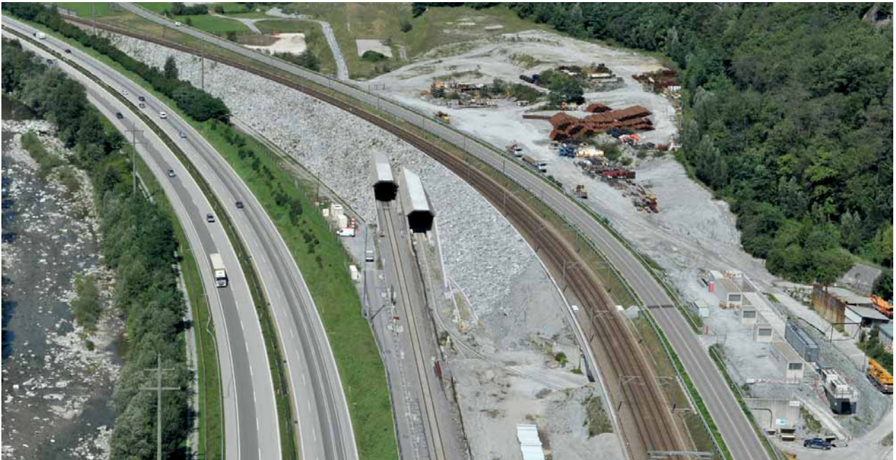
3 Südportal des Gotthard-Basistunnels in Bodio Gotthard Base Tunnel south portal at Bodio
