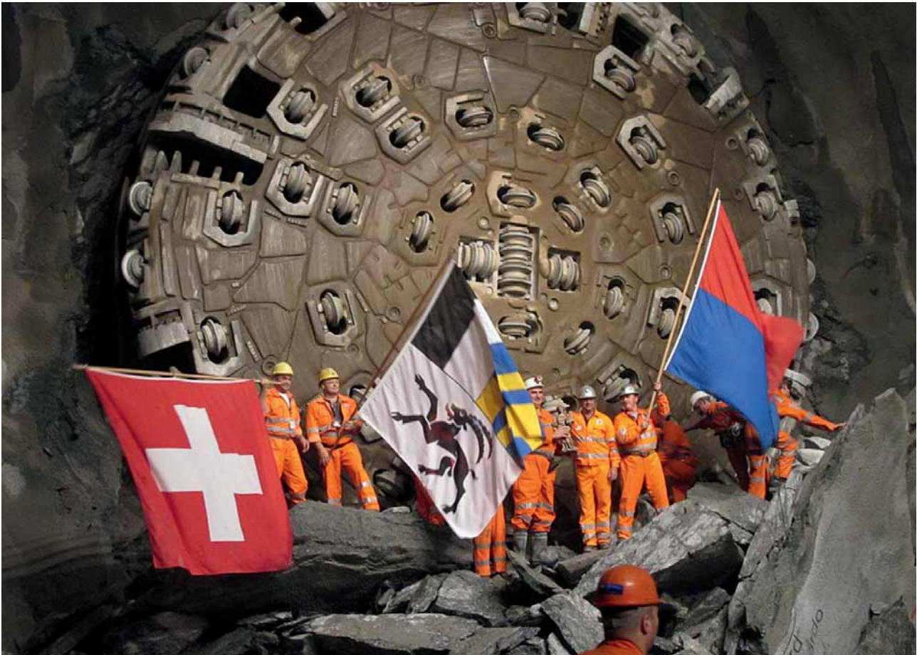
7 Hauptdurchschlag Oströhre am 15. Oktober 2010 Main breakthrough of eastern bore on October 15, 2010
