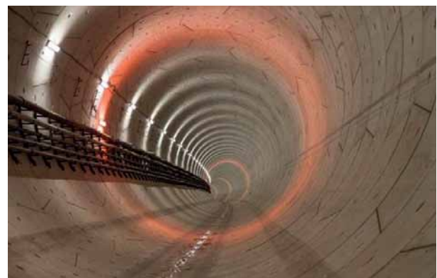
8 Vue du tunnel Nord en cours de foration View of the North tunnel during drilling
