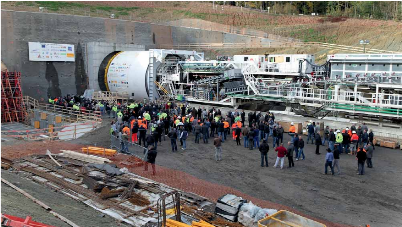
5 Tunnelier en phase de montage Tunnel boring machine during assembly
