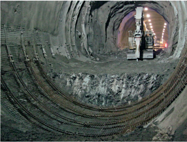
14 Section re-excitation in the North-West tunnel (Tm 0-40)
