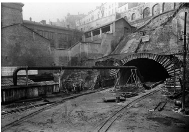
1 Percement du tunnel existant 1939 Drilling of the existing 1939 tunnel
