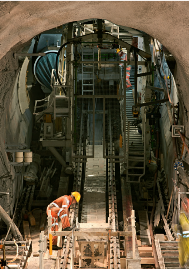
8 Tunnelbohrmaschine Druckschächte Tunnel boring machine – pressure shafts
