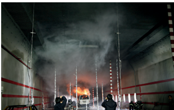
11 Experiments at the fire site of the full-scale tunnel
