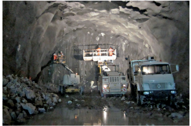
19 Front principal en cours de chargement Main rock face during charging
