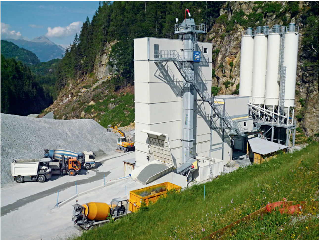
11 Betonanlage Châtelard Châtelard concrete plant
