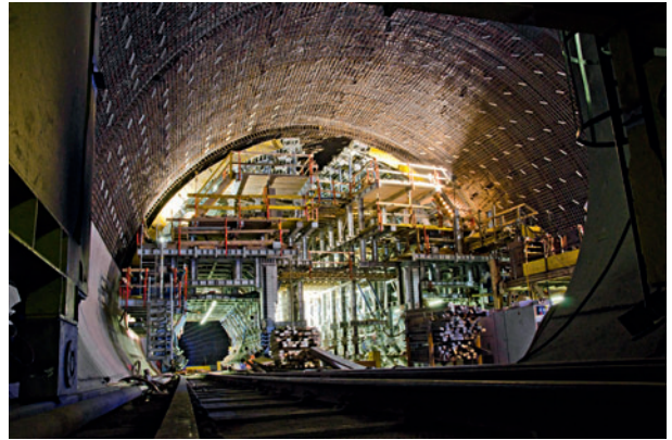
5 Innenausbau Faido, Spurwechsel Nord Faido inner lining, North crossover
