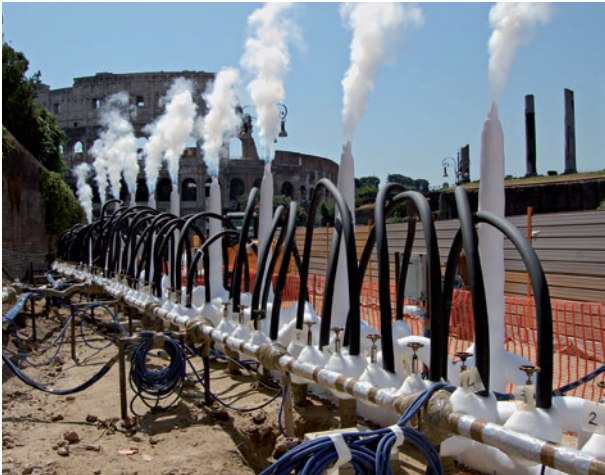
5 Ground freezing trial photo – “Via dei Fori Imperiali”
