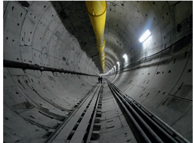
8 Primary support installed by concrete segments
