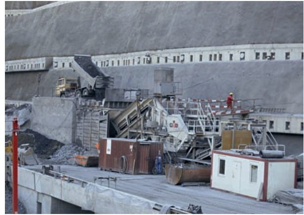
6 Backenbrecher Jaw crusher
