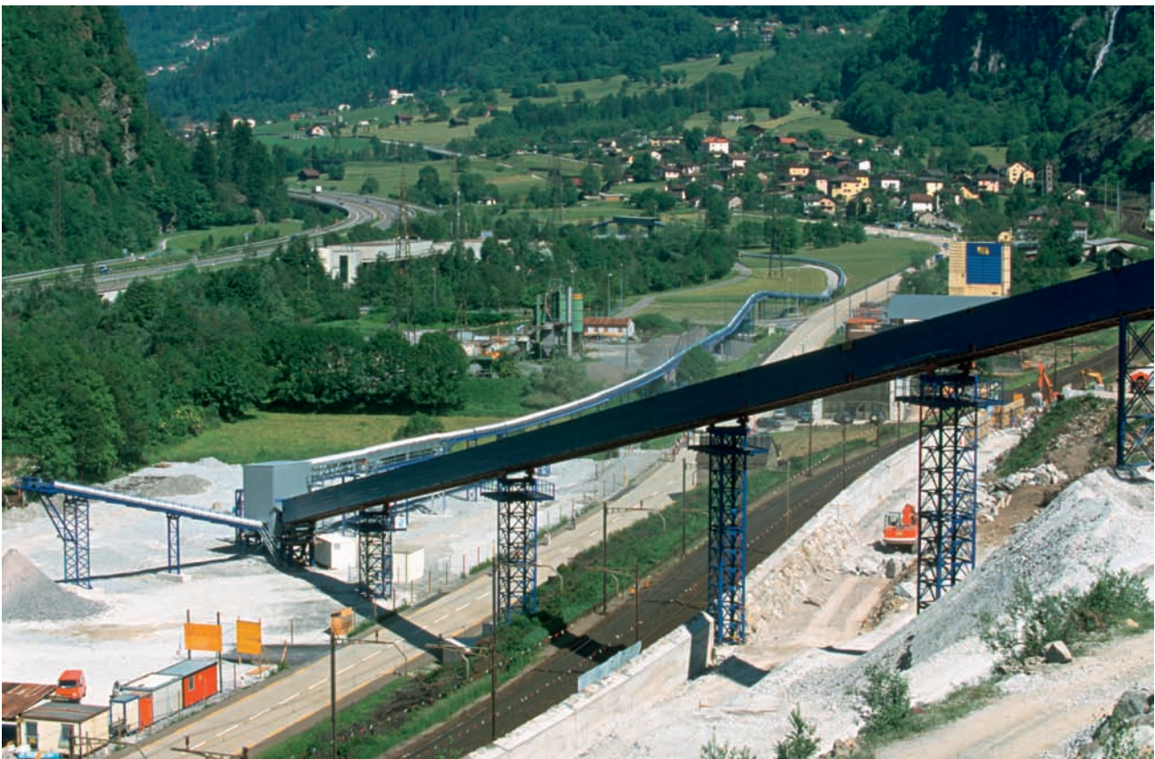
1 Deponieband Caviencia (CH) The Caviencia landfill belt (CH)
