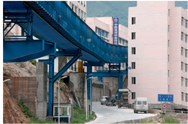
12 Bandverlauf durch Baustellencamp Jinping (CN) Routing of the belt through the site camp at Jinping (CN)
