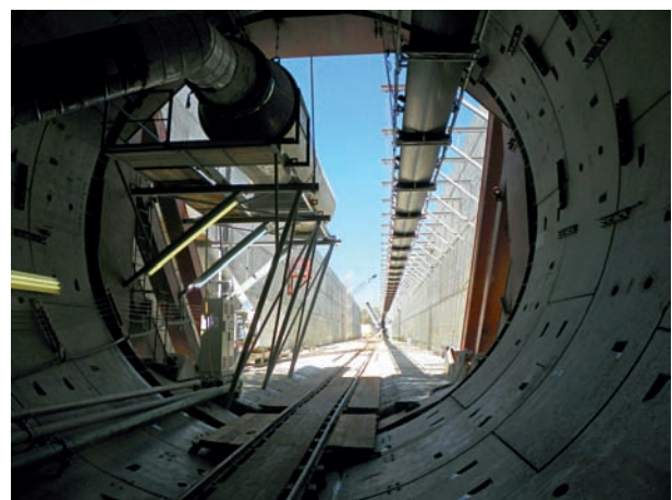
10 View of the exit canal from the tunnel
