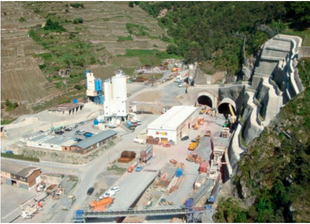
5 Installationsplatz Staldbach The Staldbach work yard
