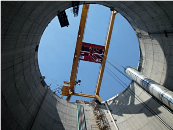
7 Upper part of Shaft 5
