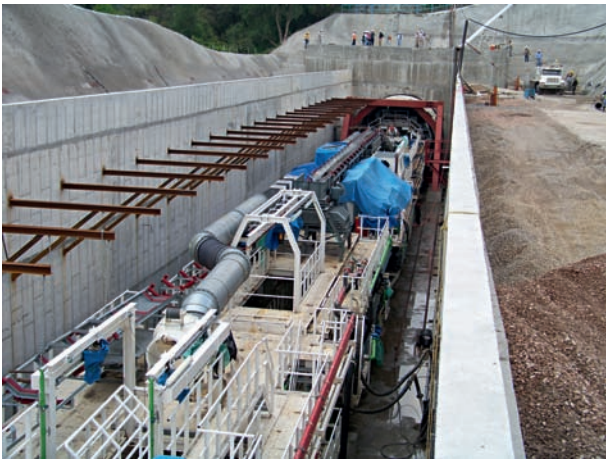
5 EPB type TBM starting the excavation at the end tunnel section
