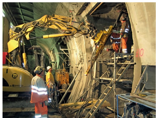
14 Ankerversetzlafette Mobile drilling carriage used for setting of rock bolts
