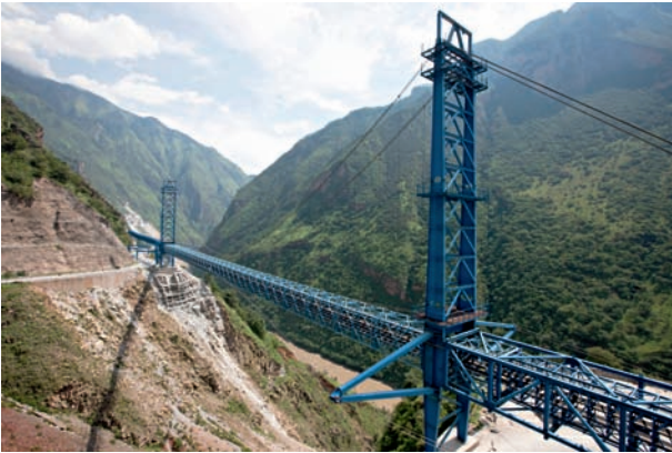
11 Hängebrücke Jinping (CN) Suspension bridge at Jinping (CN)
