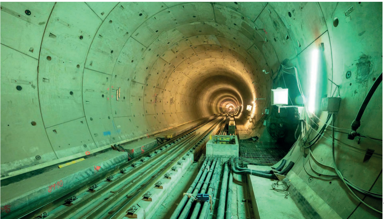
7 Constructing slab track, emergency walkway, verge
