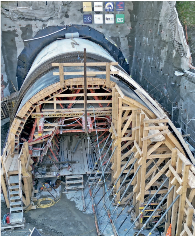
3 Start of concreting
