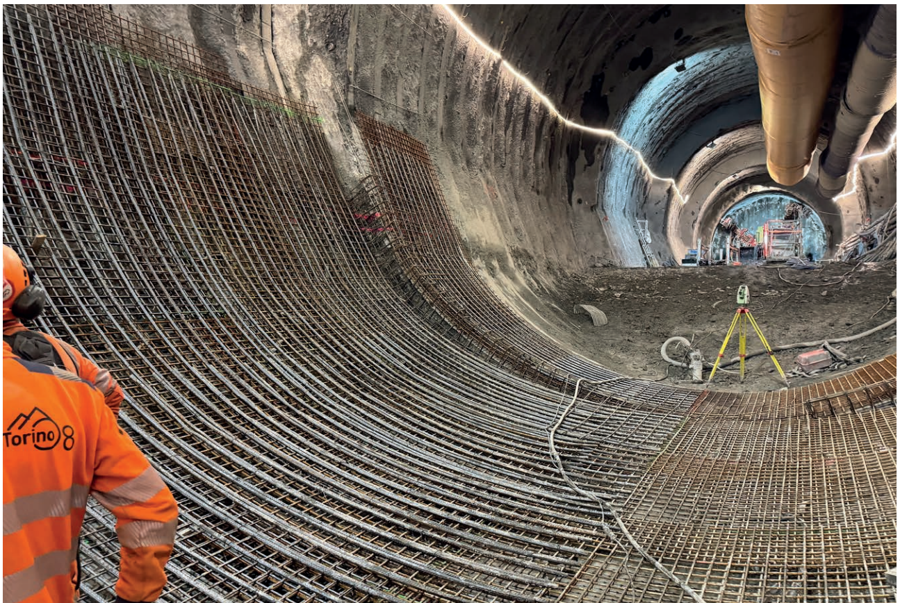
13 Installing the reinforcement invert
