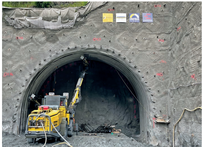
5 Drilling pipe screens in the tunnel
