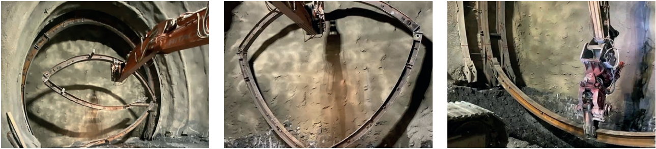
11a, b, c Automatic steel arch installation procedure
