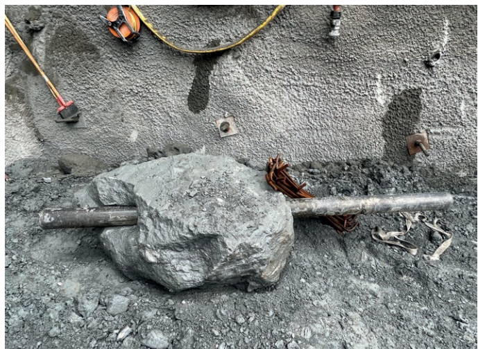
7 Boulder found in the tunnel face
