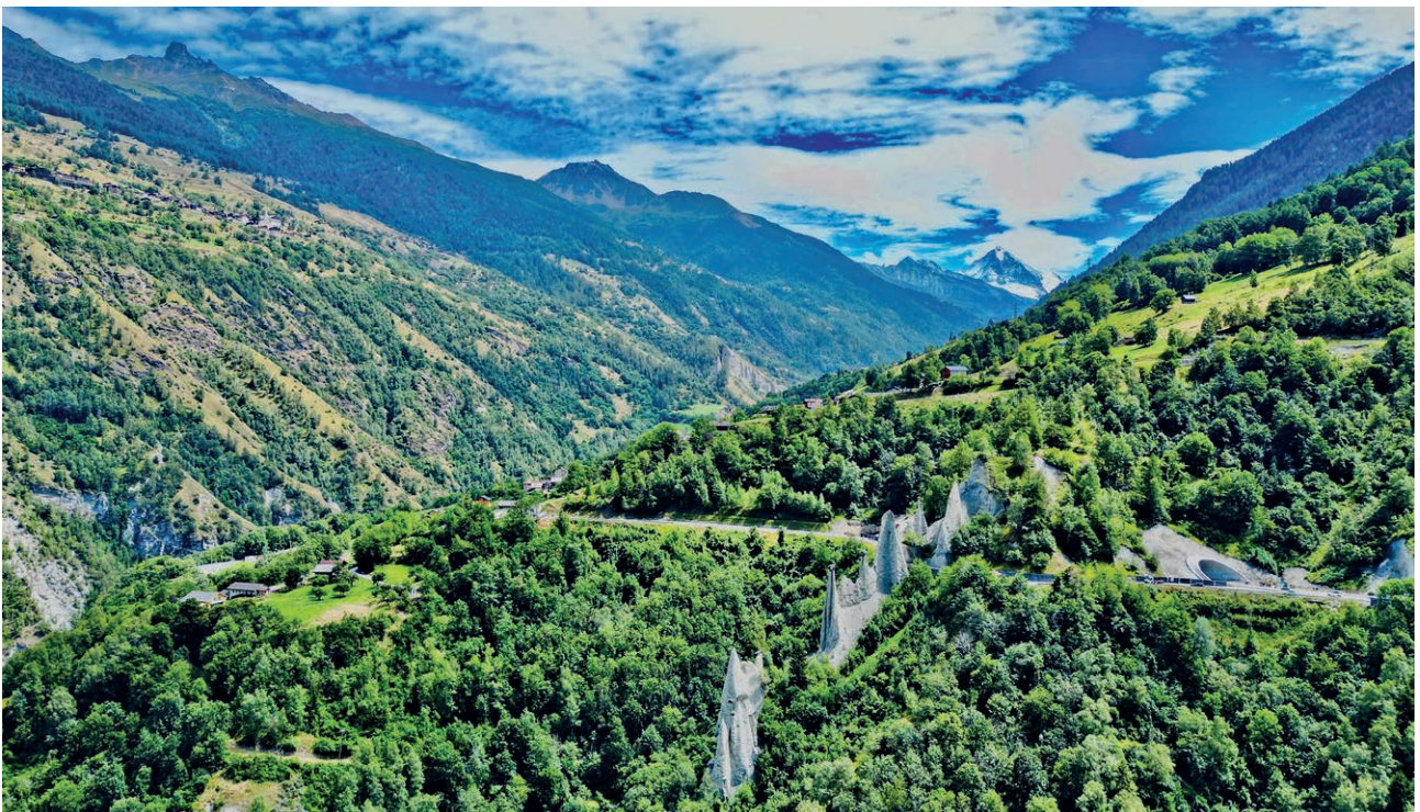
8 Completed construction work
