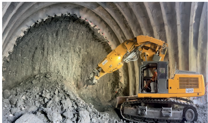
6 Excavation using a hydraulic shovel and ripper bucket
