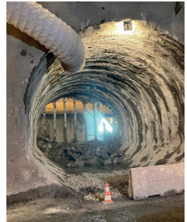
12 Breakthrough of cross-passage 2
