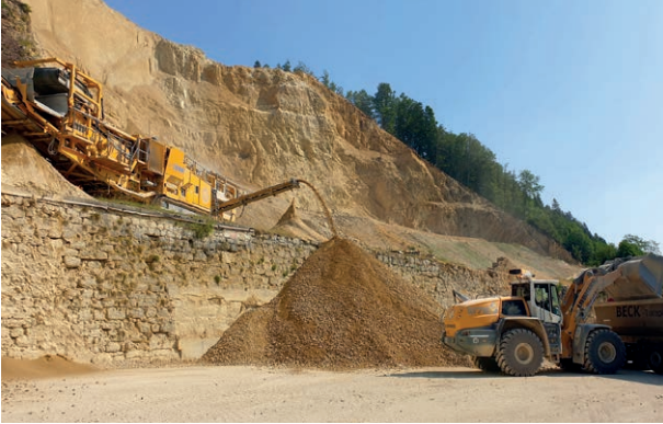
10 Le Locle bypass, stabilisation work with rock removal at the western portal
