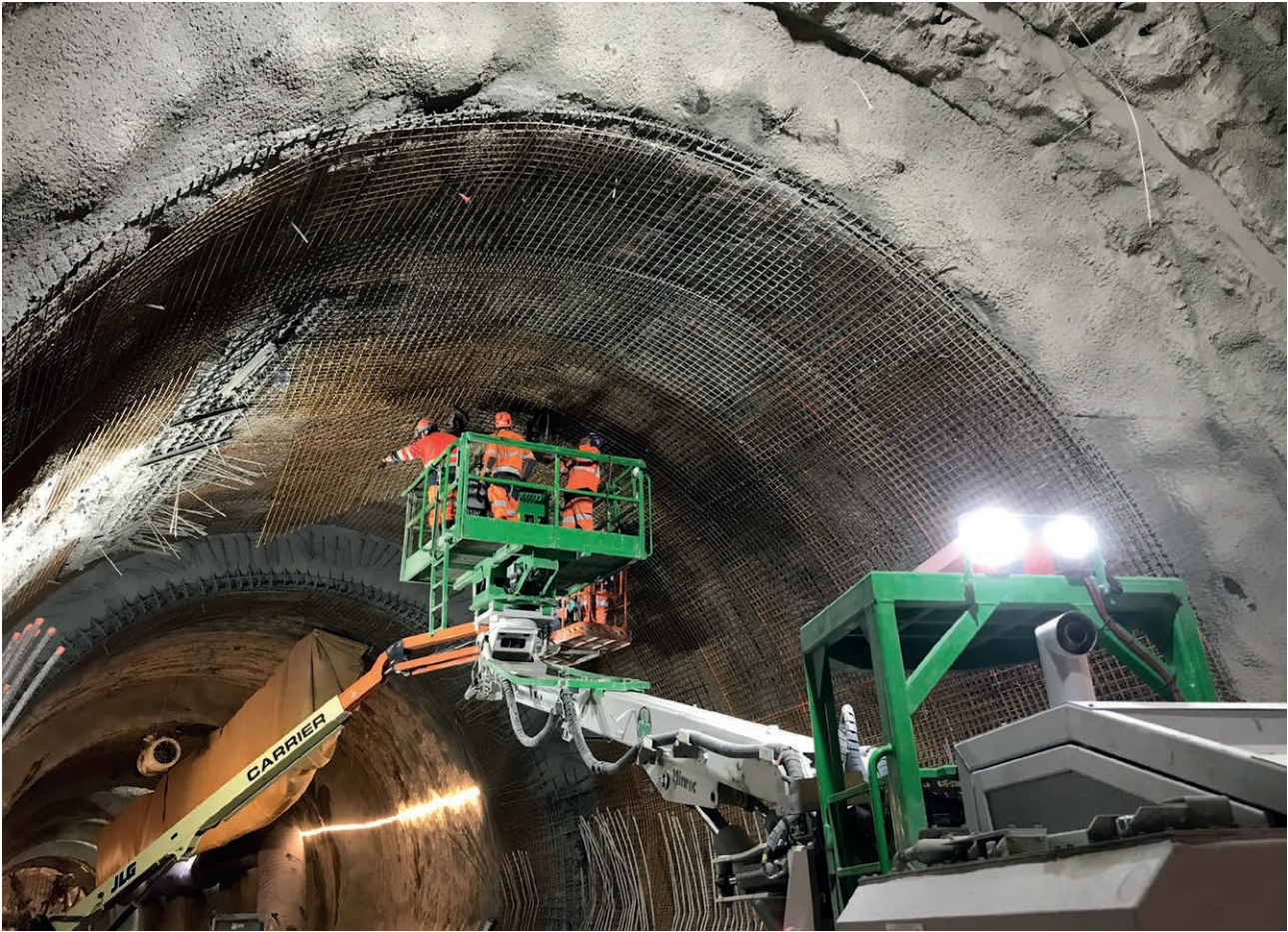
14 Installing the reinforcement top heading/crown
