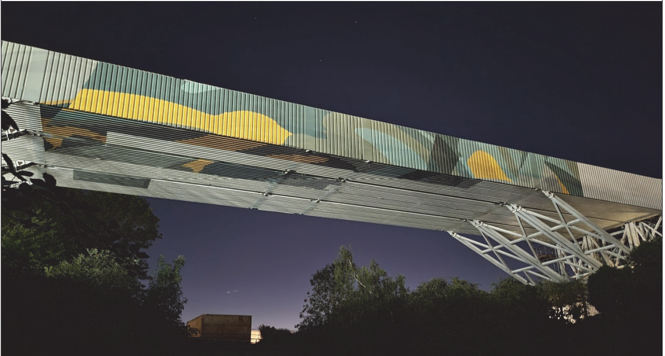
HS2-SCS High Speed London – Birmingham (United Kingdom) www.rowa-ag.ch
