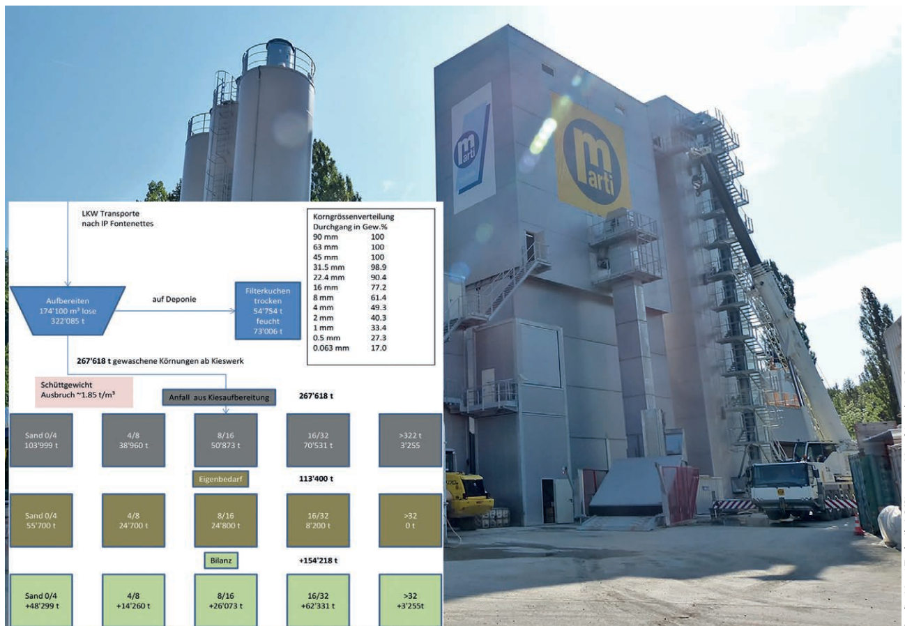
4 Tunnel de Champel (Cornavin–Annemasse). Gravel pit directly by silos in a concrete plant.
