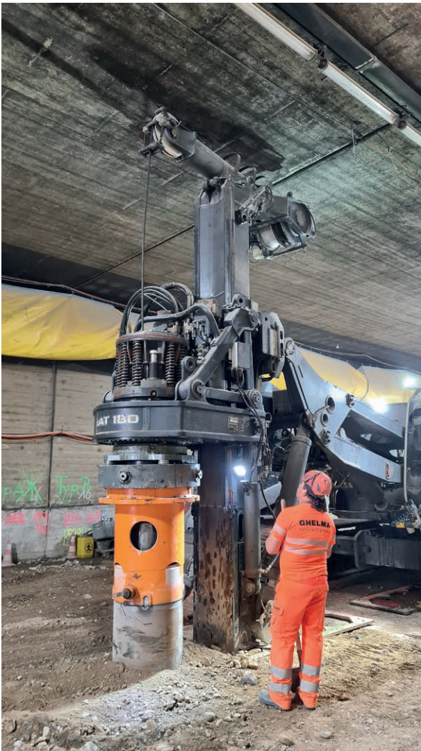
7 Drilling rig with low headroom, ARGE GUBRI/sub-contractor Ghelma AG, Civil Engineering Specialist
